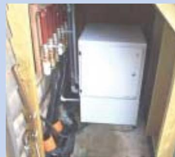
Fig 1: Picture features 8kW heat pump unit connected to the ground loops via the red manifolds. Picture courtesy of Kensa Engineering.
