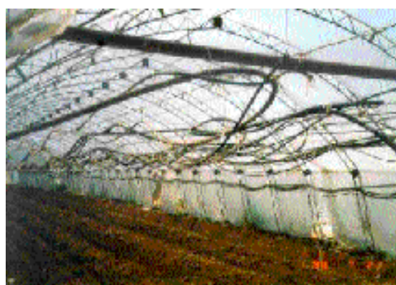
Fig.14. Characteristic parts of the “Smokvica” geothermal system: Connection lines of the wells to the central pump station; Greenhouse complex of 22,5 ha, and plastichouses complex of 10,00 ha
