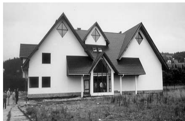
Fig. 6. A new geothermal heating plant in Bańska Niżna.
